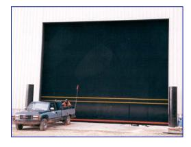
This surface mine shop is designed to maintain a fleet of 290-ton haul trucks and various other mining equipment. There are three service bays and one wash bay.
